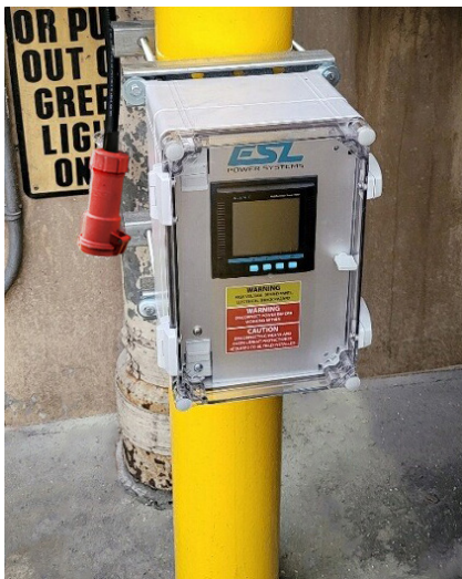
30A 600VAC eTRUconnect Power Meter Panel Item #: 1423-37
