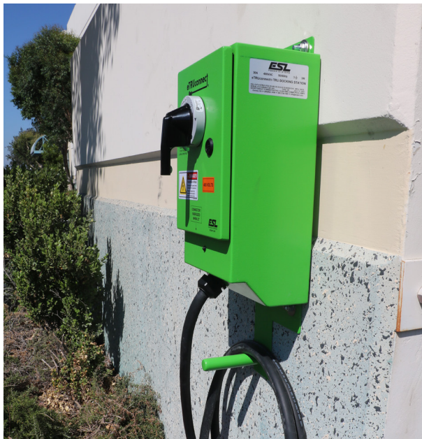
30A 480VAC eTRUconnect V2 PS Series with cord hanger
