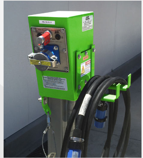
50A 208VAC eTRUconnect Power Station MC Series
