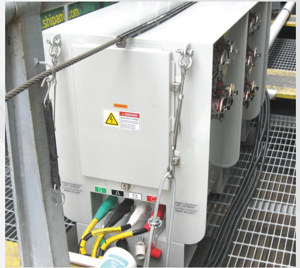
10-Gang Modular RSU Assembly ESL Series: 3500-16
