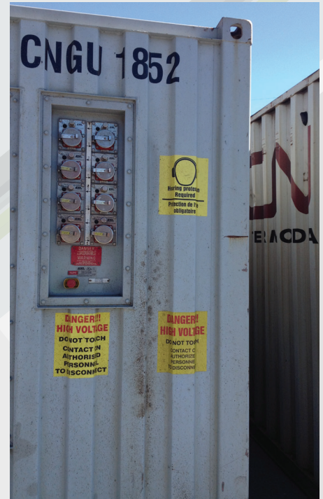
8-Gang Power Pack Assembly ESL Series: 2202-75D
