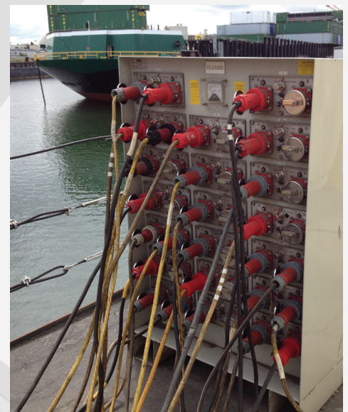
20-Gang Modular RSU Assembly ESL Series: 3500-02
