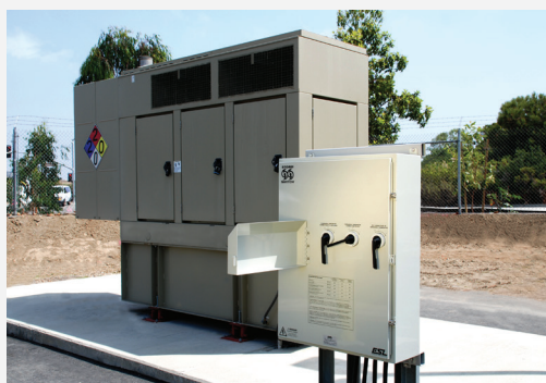
400A TripleSwitch™ ESL Series: 3140-10V
