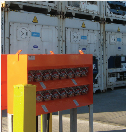
16-Gang Free Standing Assembly ESL Series: 2217-56B
