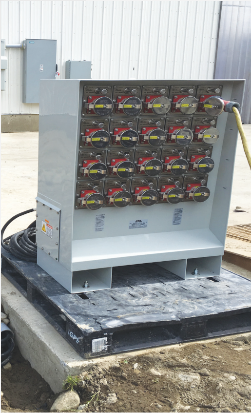
20-Gang Portable Distribution Tree ESL Series: 2280-95FNW
