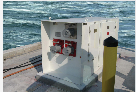
Multi-Gang Shore Power & Communication ESL Series: 5200-47-ST2
