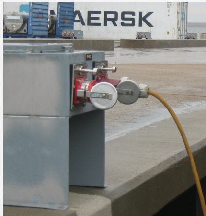
2-Gang Pedestal Mount Assembly ESL Series: 2209-26
