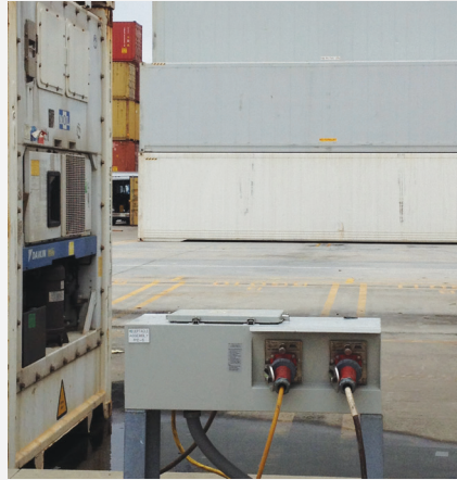
2-Gang Pedestal Mount Assembly ESL Series: 2220-78
