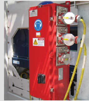
3-Gang Rack Mount Assembly ESL Series: 2222-55
