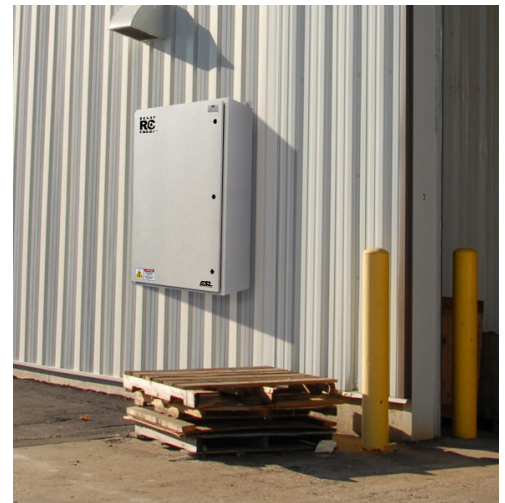
400A 480VAC Automatic Transfer Switch with Cams
