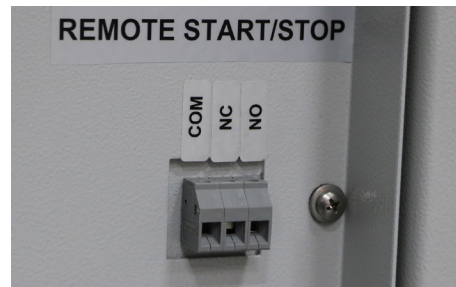
Remote start/stop connections
